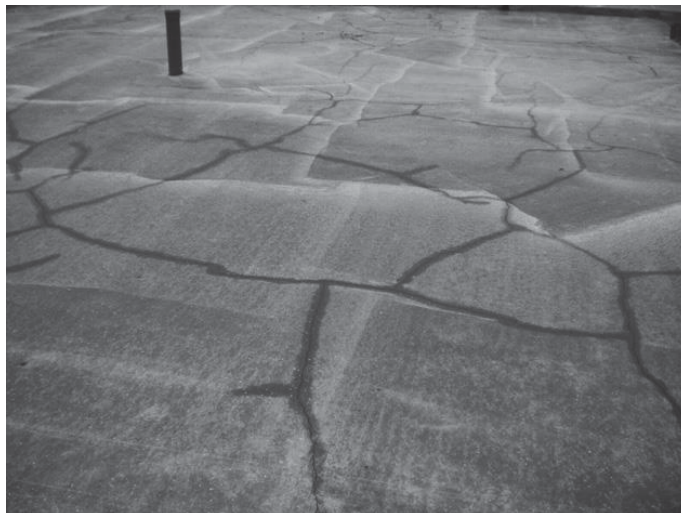
Figure 1.1 - Plastic shrinkage cracking at concrete surface from Slowik, et al. (2008).
